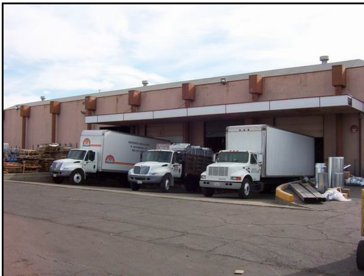
Figure 9. Loading Docks with an Overhang to Prevent Material Contact with Stormwater.
